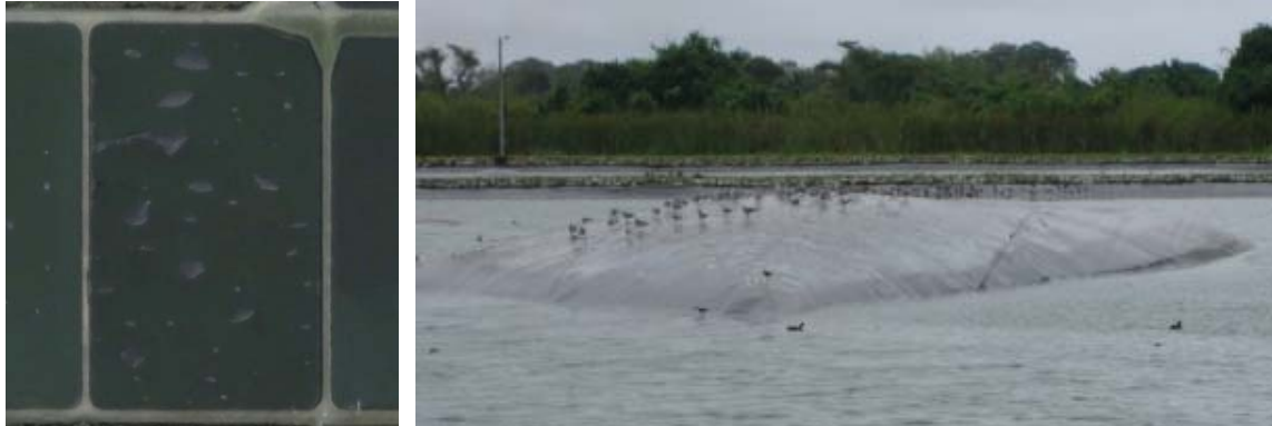
Figure 4-1: Geoliner Failure at Puerto Cortes: A) Satellite View, B) Photographed with Nesting Birds Source: A) Google Earth and B) the Author
